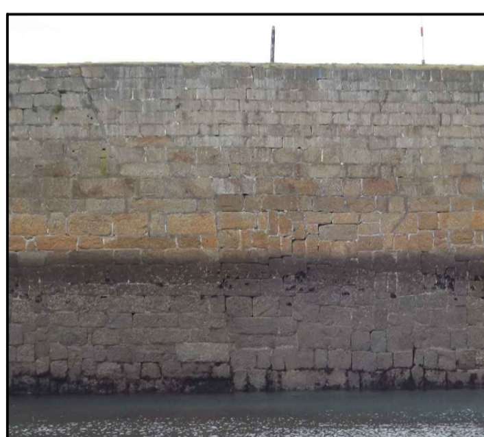
Photo 21 - Northern Section of the South Pier 2013 RHDHV Inspection
