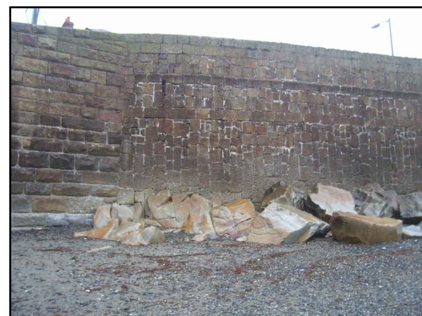
Photo 5 South Pier Protected by Rock Armour 2013 RHDHV Inspection
