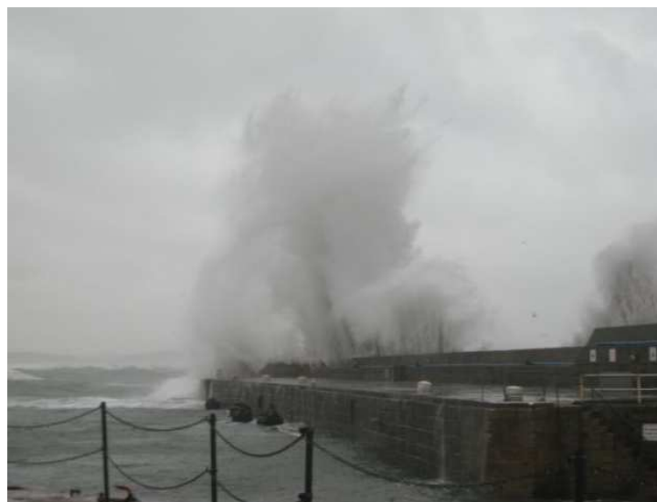
Photo 2 – Wave Overtopping at the Lighthouse Pier (Courtesy Dave Simpson, Cornwall Council)
