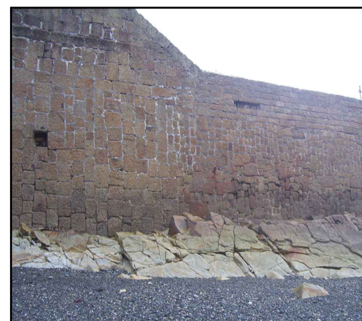
Photo 6 - South Pier Protected by Rock Outcrop 2013 RHDHV Inspection
