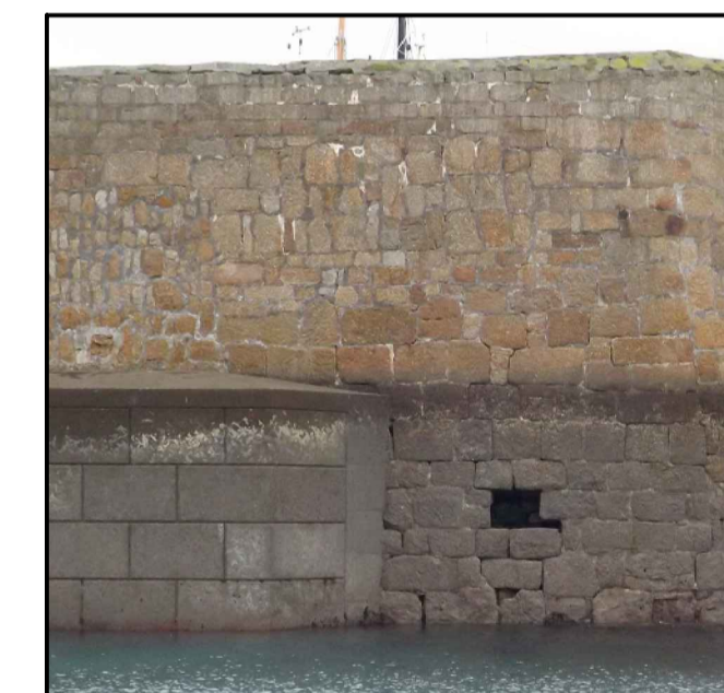
Photo 8 - South Pier Right of Concrete Build-out 2013 RHDHV Inspection
