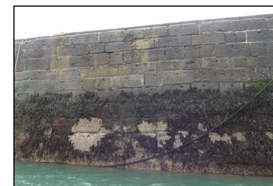
Photo 25 - Northern Face of the Lighthouse Pier 2004 Hyder Report
