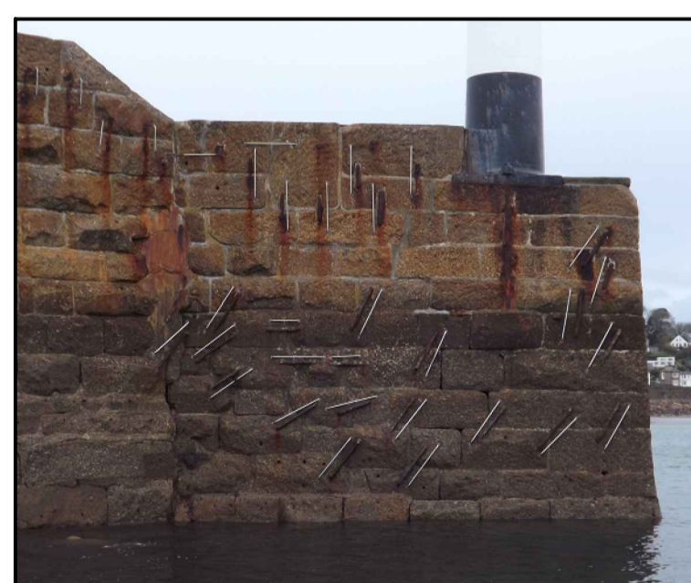
Photo 23 Western Section of the Lighthouse Pier (Southern Face) 2013 RHDHV Inspection
